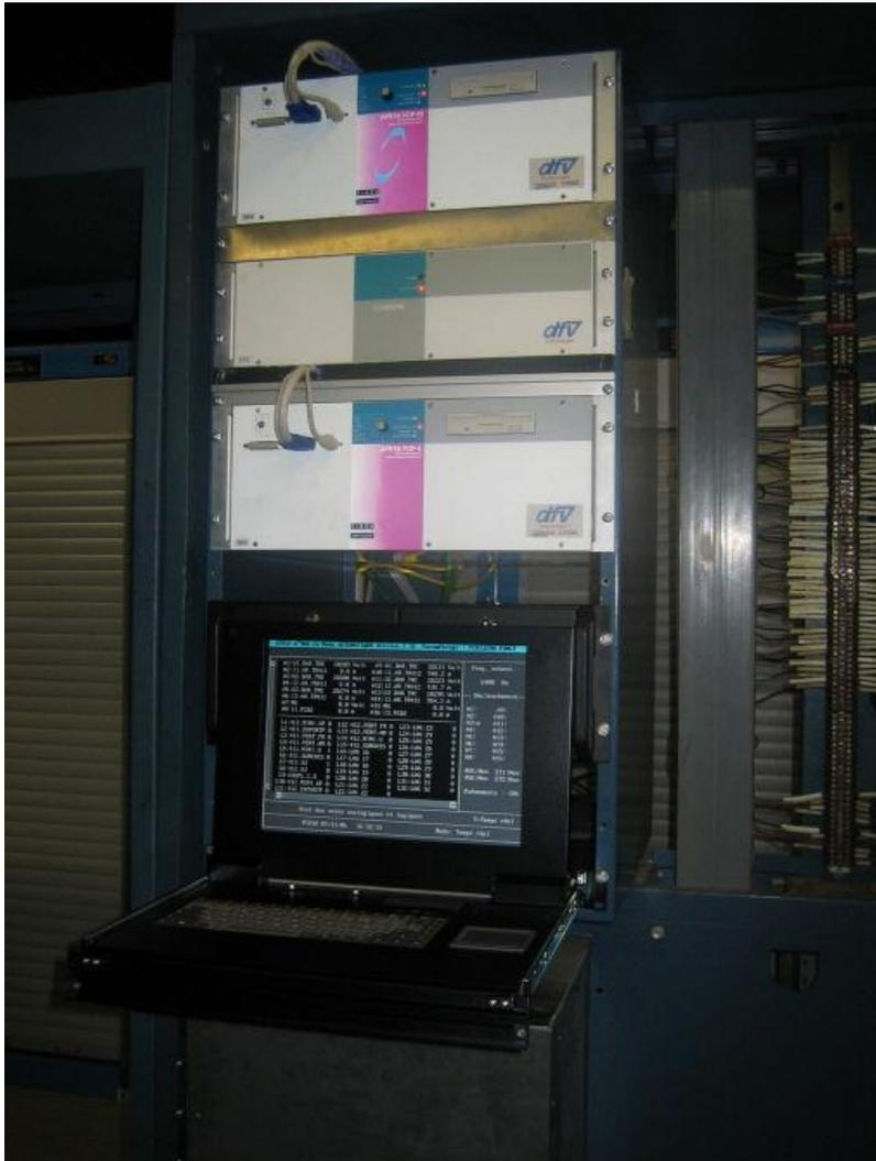
Digital Fault Recorder mounted in a 225kV station.
